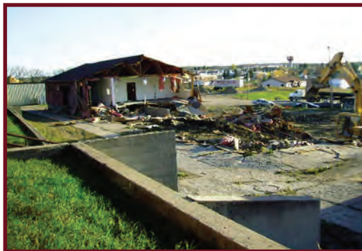
Modular unit demolition
